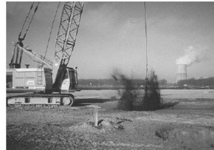
Figure 2. Compaction of deposited waste by dynamic consolidation
